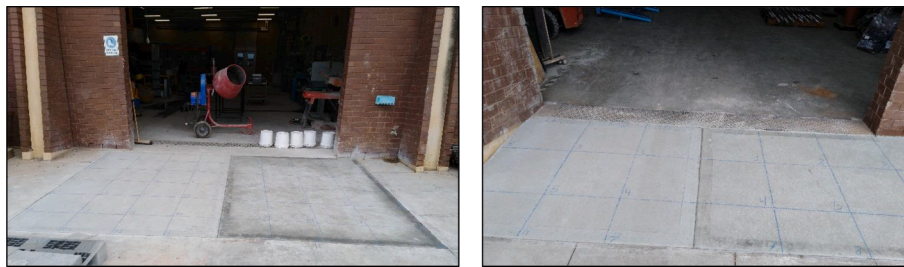
Fig. 6. The ground slab after casting and surface finishing.
