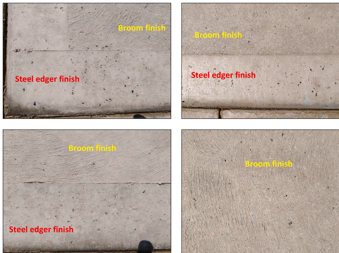
Fig. 23. Surface of CRC ground slabs at different locations.
