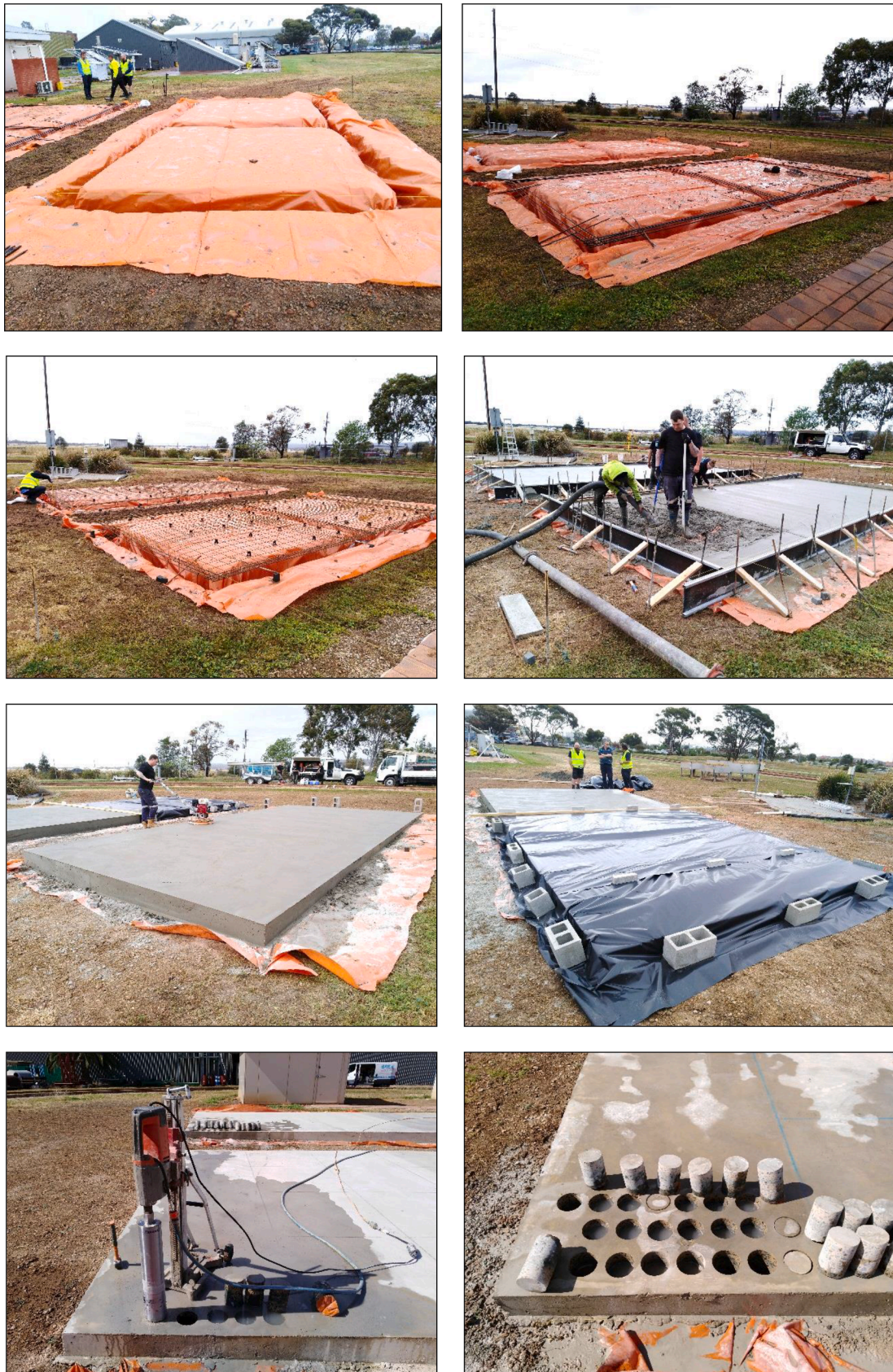
Fig. 3. Residential slab casting, curing, and coring.
