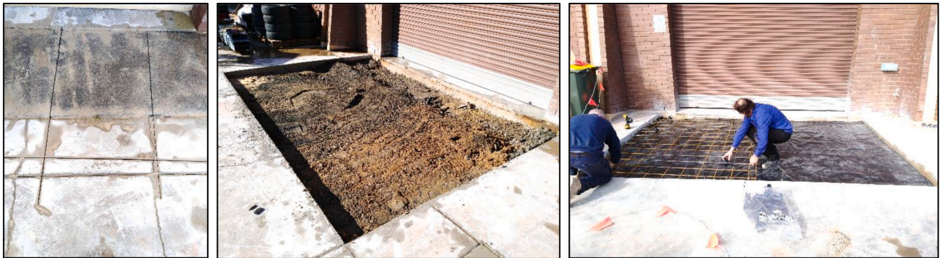
Fig. 5. Removing old ground slab and preparing for new replacement.
